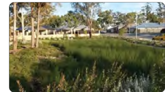
Vegetated drainage swale.
