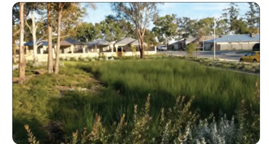
Vegetated drainage swale.
