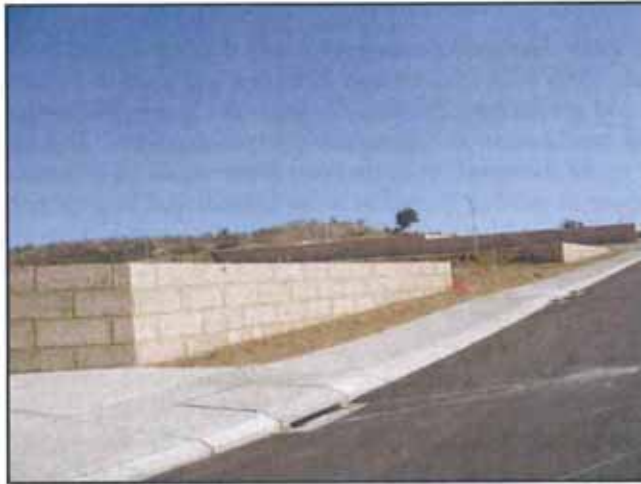
(Left) Example of terraced style retaining to create level building sites.
