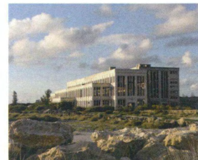
Figure 21_The South Fremantle Power Station
