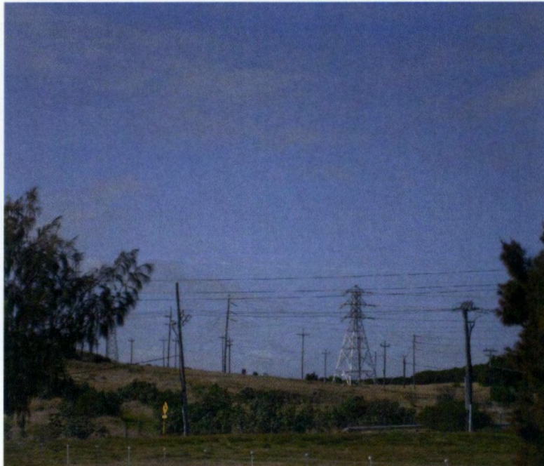
Figure 24_Existing Infrastructure of the Cockburn Coast
