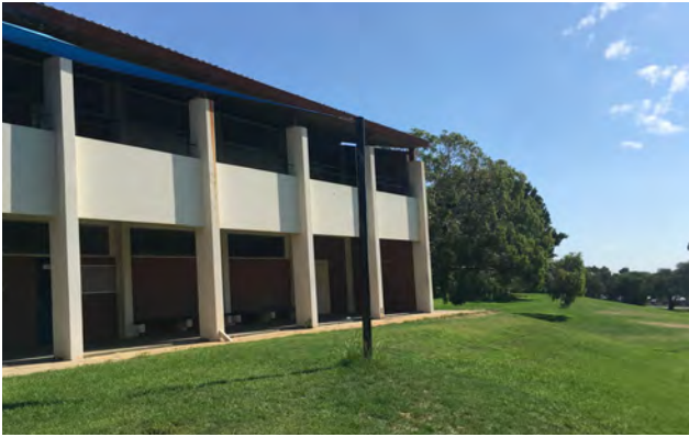
Existing built form/landscape interface
