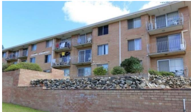
Figure 22. Glendower Way, Spearwood – 24 single bedroom apartments
