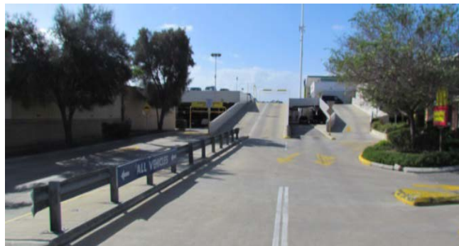
Figure 14. Ramp from Rockingham Road
